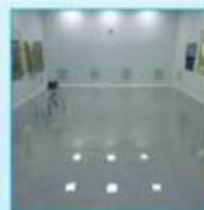
Class-1000 Clean Room
