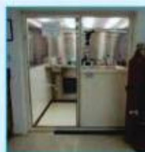
Class-100 Clean Room
