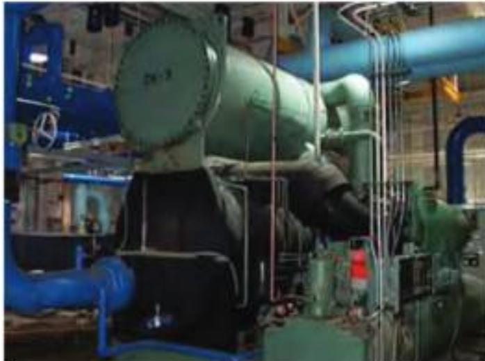
Fig.5 Typical centrifugal chiller unit
